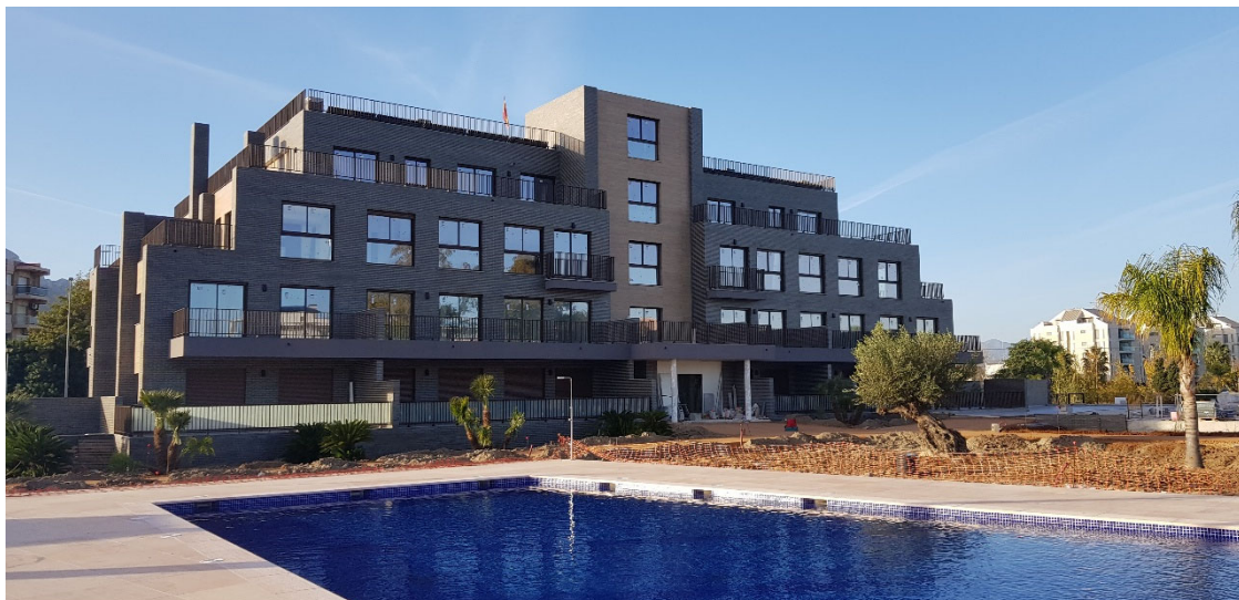
Las Lomas de Dénia Residential Complex, Block 2
