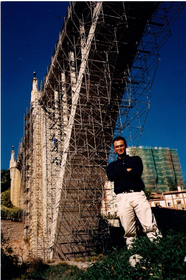
Old Viaduct of Teruel, 1996
