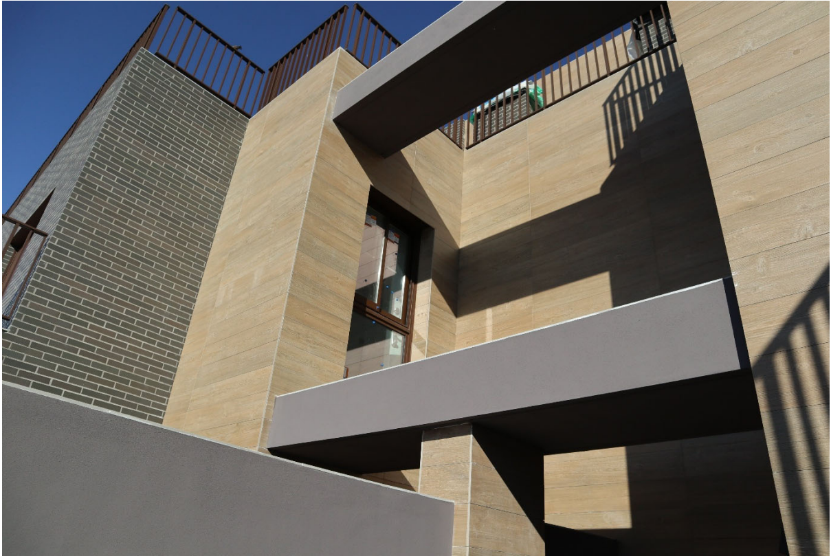
Las Lomas de Dénia Residential Complex, Block 2
