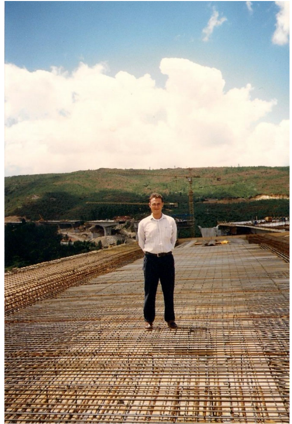
Coura Bridge, Portugal, 1997
